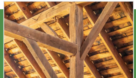
Detailed view of framing showing mortise and tenon joints.
