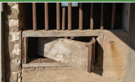
The box stalls feature a unique rotating feeding tray.
