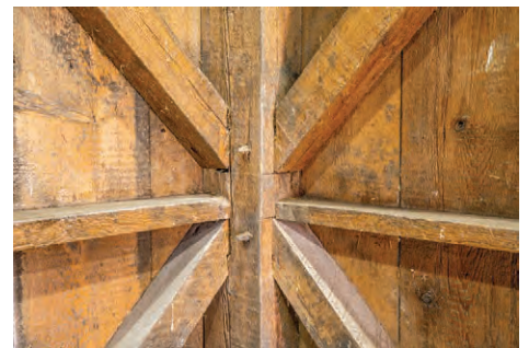
The framing and wooden pegged mortise and tenon joints come together like a work of art.
