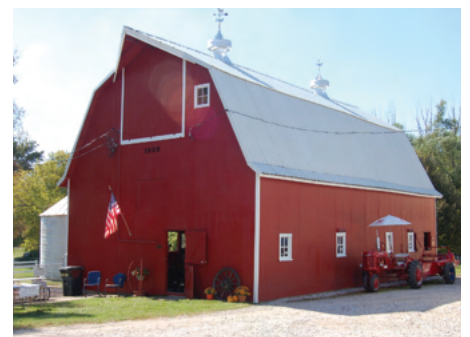
Rimathe Family Barn, 51349 Highway 210, Slater (Story County)
