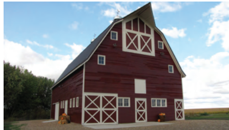
Johnson Barn, 4594 Vine Ave, Sutherland (O'Brien County)
