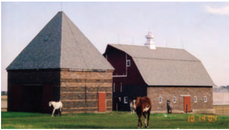
Ferguson Barn, 40415 130th Avenue, Laurens (Pocahontas County)
