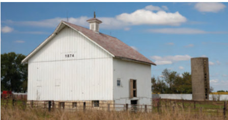
Gillespie Barn, 1257 Highway IA 92, Winterset (Madison County)
