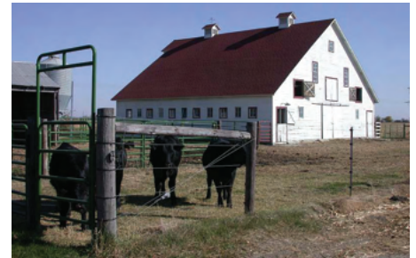
Belfrage Barn, 2410 Port Neal Road, Sergeant Bluff (Woodbury County)
