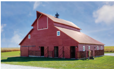
Lundy Barn, 11450 680th Avenue, Zearing (Story County)
