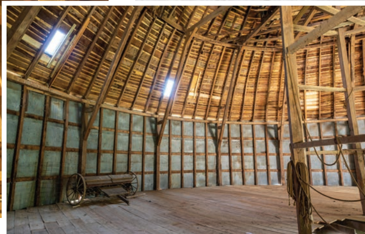
As part of the restoration, a major portion of the haymow floor was replaced.
