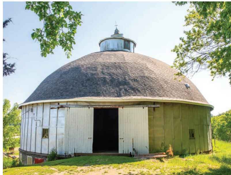
The bank barn design allowed for wagons to be pulled through two sets of doors on the upper level with livestock access to the lower level. Photo by Dave Austin.
