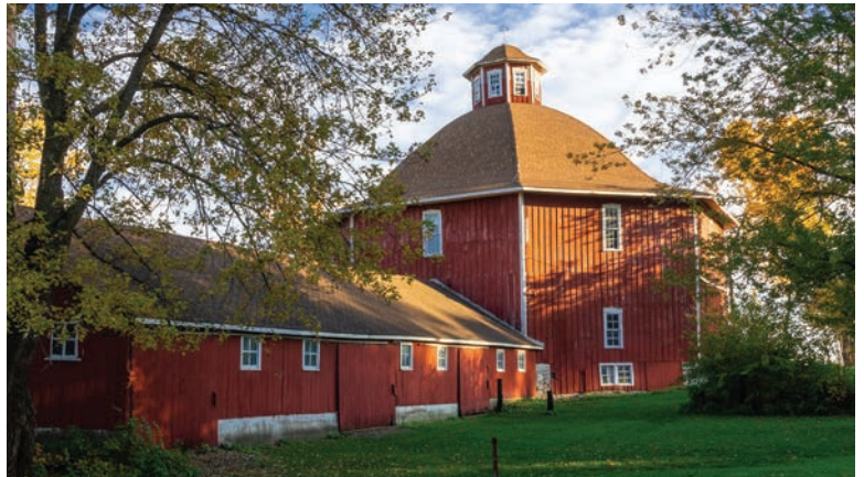
The Secrest Barn was built first, with cattle shed being attached later, followed by an addition of a clay tile silo.
