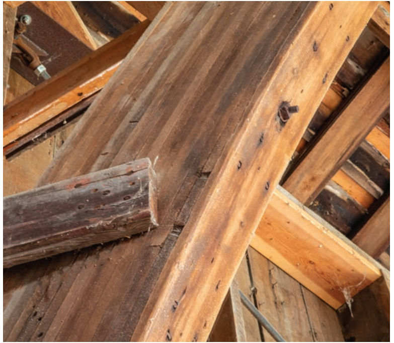
Close-up view of one of the laminate ribs formed from 18 1-inch thick boards providing the strength to support the barn's roof.
