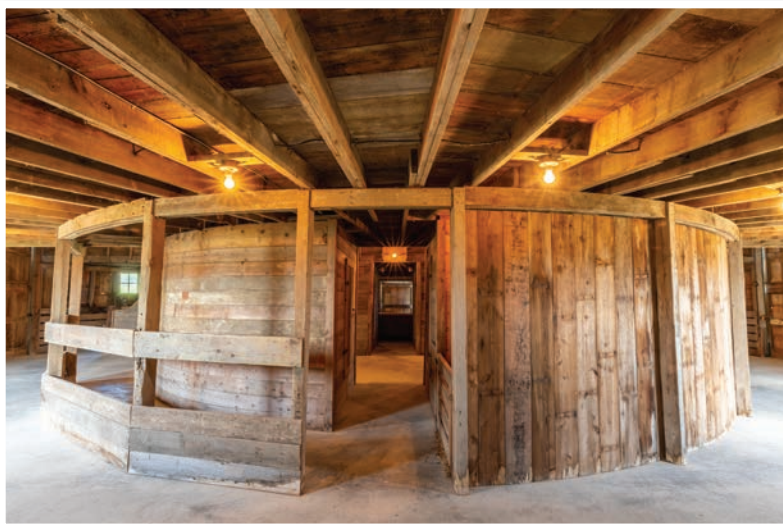
The pie-shaped grain storage bins are formed by the intersecting hallways.
