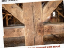
Mortise and tenon joints secured with wood pegs in the haymow.
