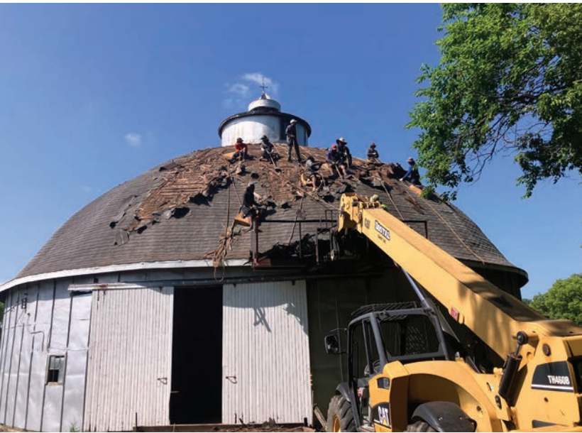
Roofers tackling the challenging job of removing the old shingles. Photo by Kari Friedlein
