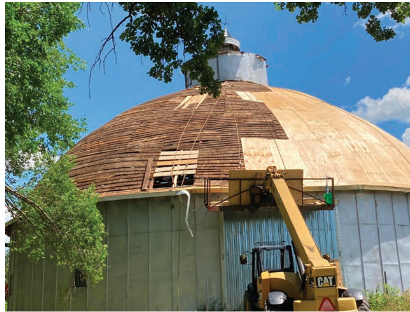
The roof replacement required over 120 4x8 sheets of plywood sheathing. Photo by Kari Friedlein
