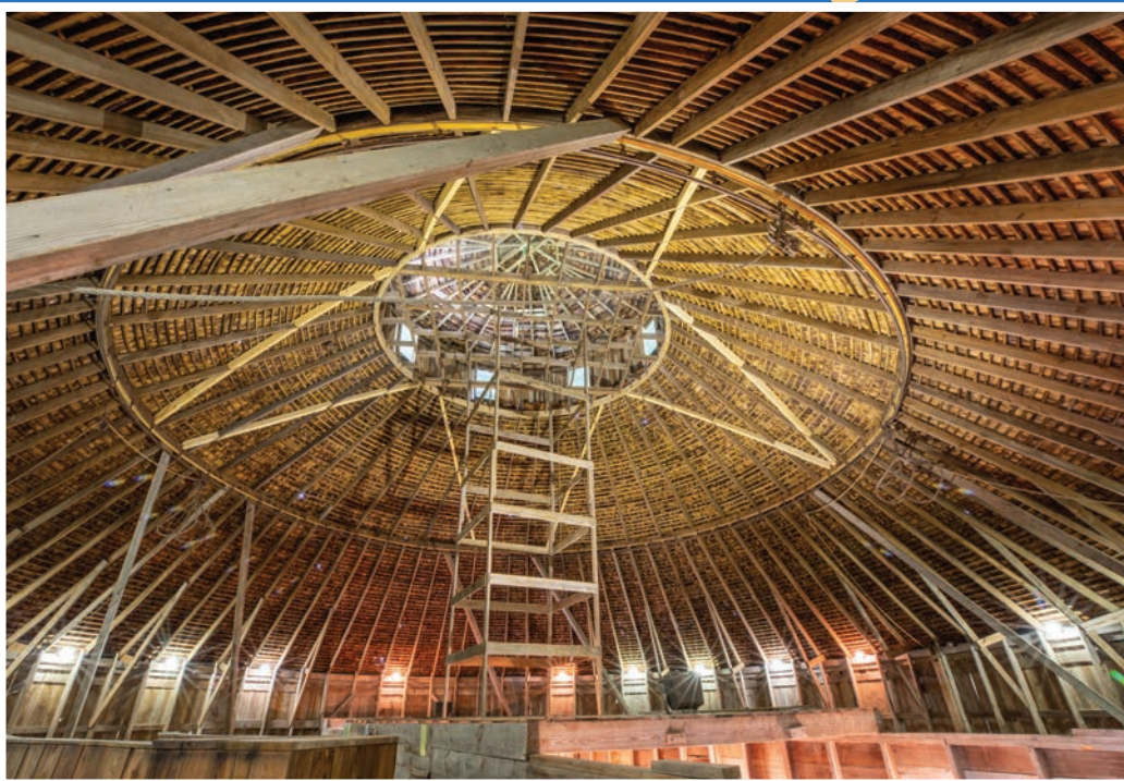
Haymow view showing the full-circle Louden track and hay fork carrier system for filling the barn with loose hay.
