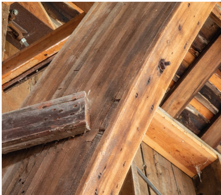
Close-up view of one of the laminate ribs formed from 18 1-inch thick boards providing the strength to support the barn's roof.
