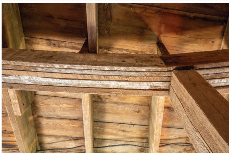
The laminated mid-span ring beam is created from six one-inch boards bent nailed into the circular shape.
