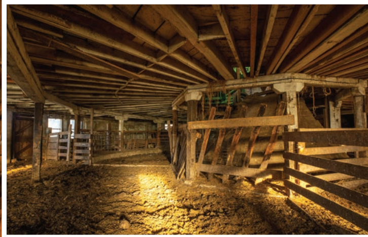
A view of the first level before restoration showing the flooring joists supported by the ring beams. Photo by Dave Austin
