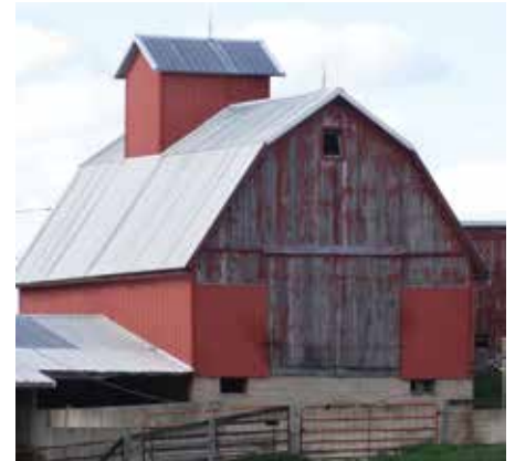
Figure 6: This corn crib was built on a limestone basement with an earthen ramp on the other end. The Aarik Deering farm in Allamakee Co., IA.
