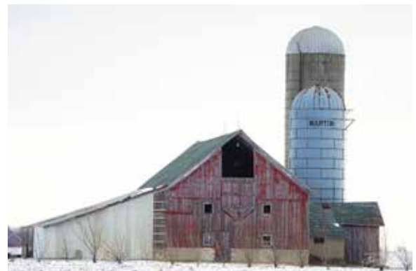
A steel panel silo standing in front of a concrete stave silo in Sumner, IA (photo by Ron Scholten).
