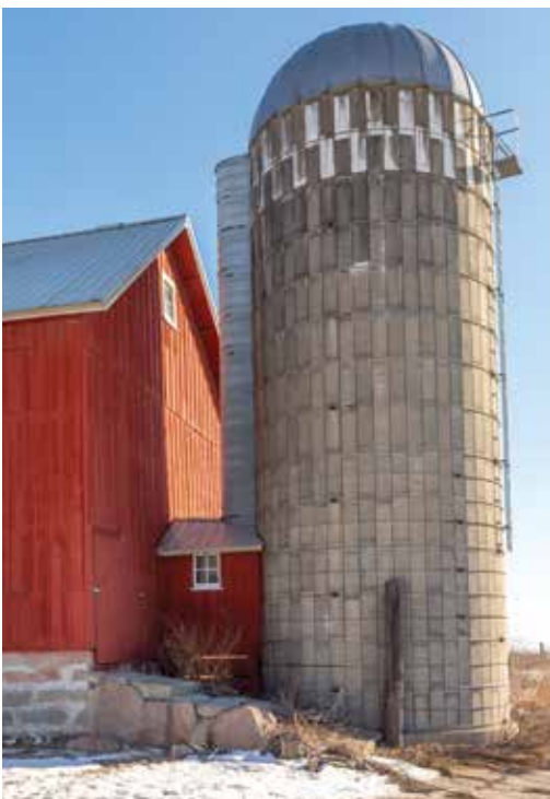
A concrete stave silo on the Jensen farm in Waverly. Concrete staves become the most common silo construction material due to their durability and low cost.
