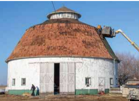
Work crew removing 3 layers of old roofing and installing the new cedar roof.
