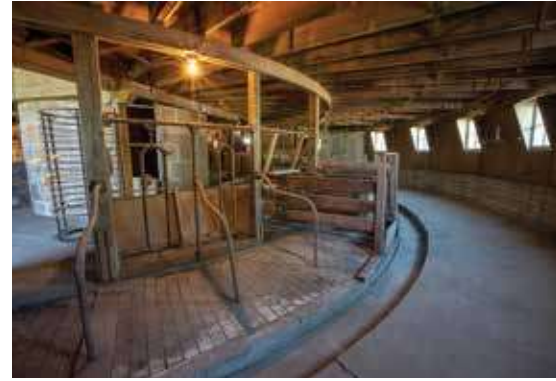
View of the dairy stanchions and hog farrowing stalls on the ground floor.
