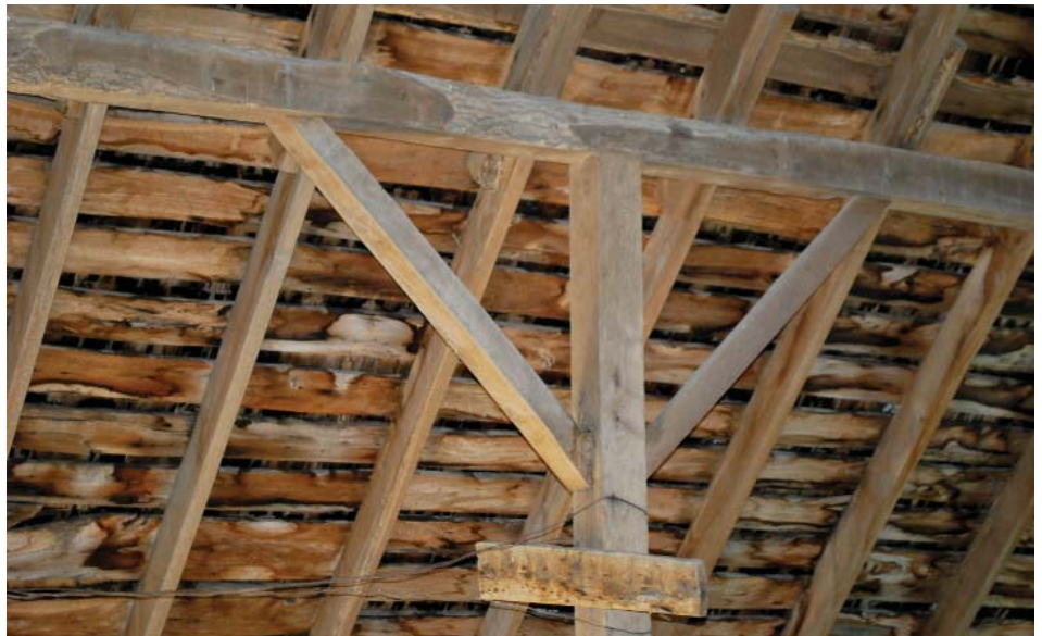
Smith barn, interior
