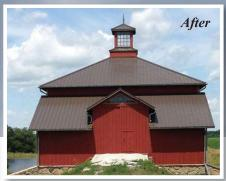
With the foundation repaired or shored, and the frame repaired or shored, we move to the roof. If the roof is in need of repair or replacement, this becomes the top priority. If there is a roof back on the building work to the foundation, and the frame can occur at a later date if needed.
